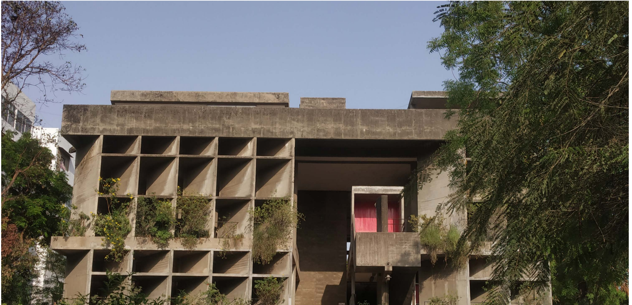
Le Corbusier / The Mill Owners' Association Building, Ahmedabad, India, 1954. (photo: Akshaya Ramakrishnan)
