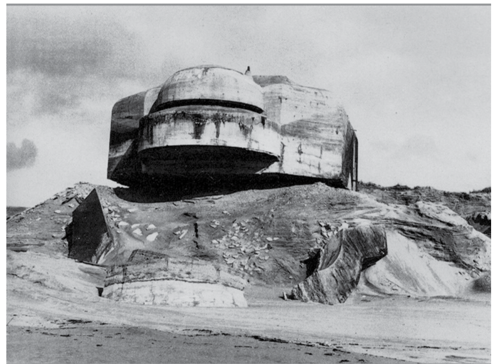
A German Bunker of the Atlantic Wall, Bretagne, France. (photo: Paul Virilio)
