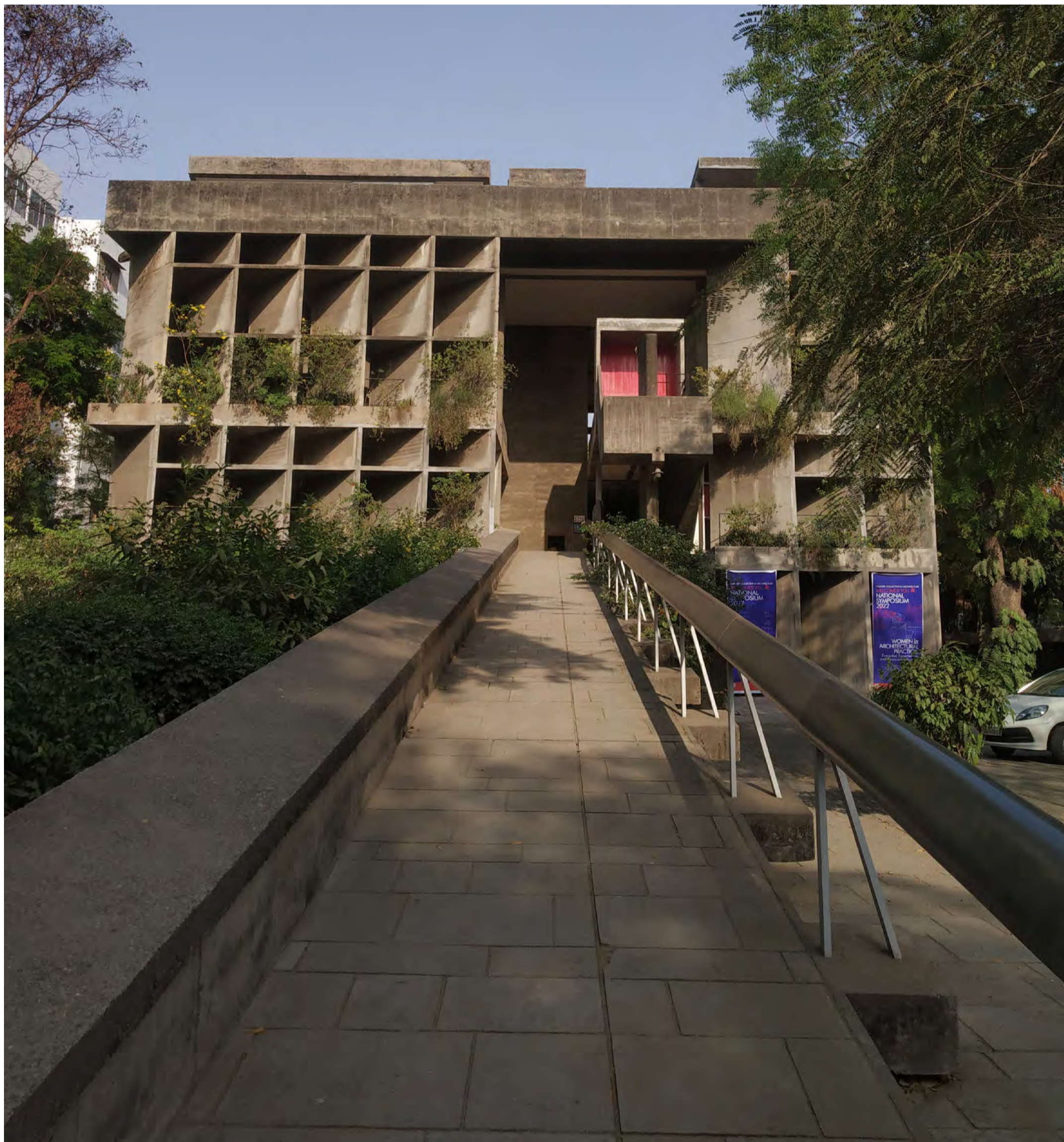
Le Corbusier / The Mill Owners' Association Building, Ahmedabad, India, 1954. (photo: Akshaya Ramakrishnan)
