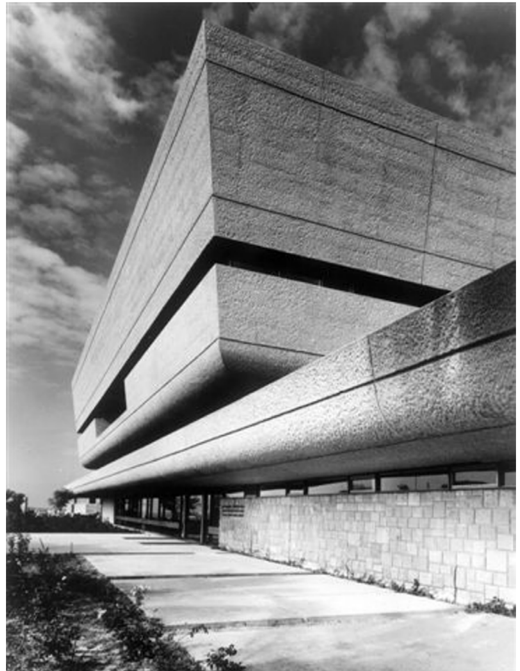
Surasky Library, Tel Aviv University . Architects: Nadler, Nadler, Bixon
