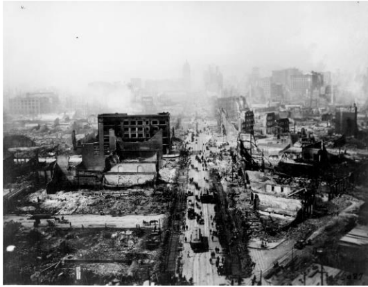
San Francisco, 1906 Earthquake
